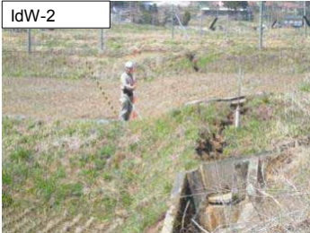
IdW-2 Look toward north. West side trace in 2 lines of flexures. Vertical displacement was 60cm.
