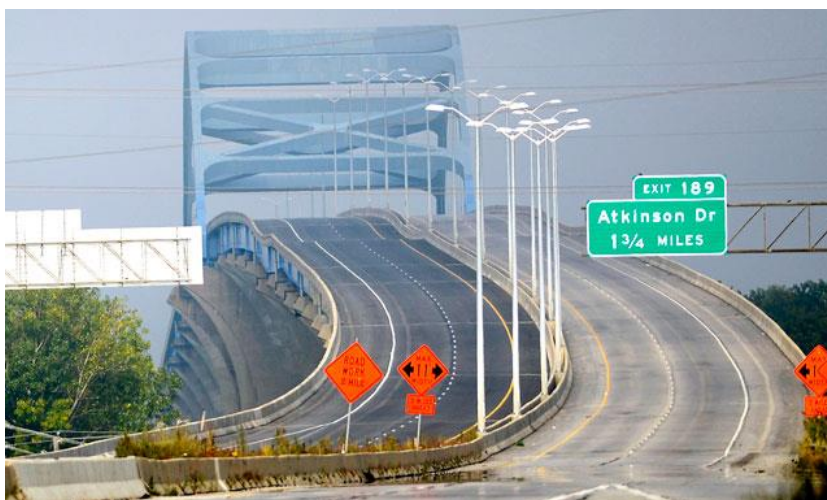
(橋脚の沈下状況)
