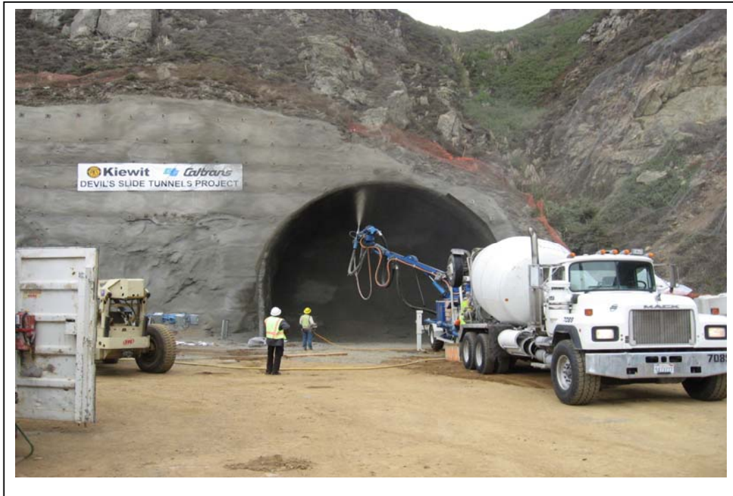
(Devil's Slide Tunnel Project 現場見学)
